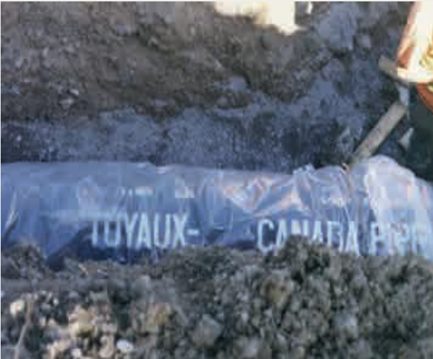
Ductile Iron Pipe installed with 8 mil polyethylene encasement in aggressive soil conditions.
