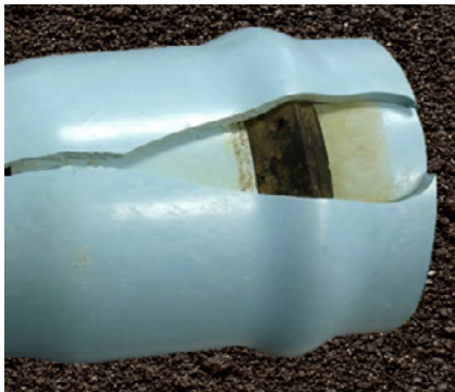
Typical splitting of PVC pipe bell from over-insertion of PVC spigot end during joint assembly.
