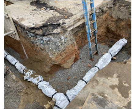
DI pipe and fittings easily and reliably protected in corrosive environments with V-Bio encasement.
