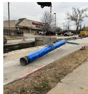
annual water main breaks. KC Water is currently replacing a two-mile section of 16" diameter cast iron main with 16" diameter zinc-coated Ductile iron pipe wrapped in polyethylene encasement. Work on this project segment began in late 2023 and is scheduled to wrap up in
